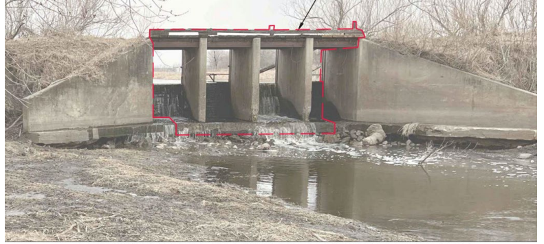
LOOKING WEST AT EXISTING LOWER STRUCTURE
