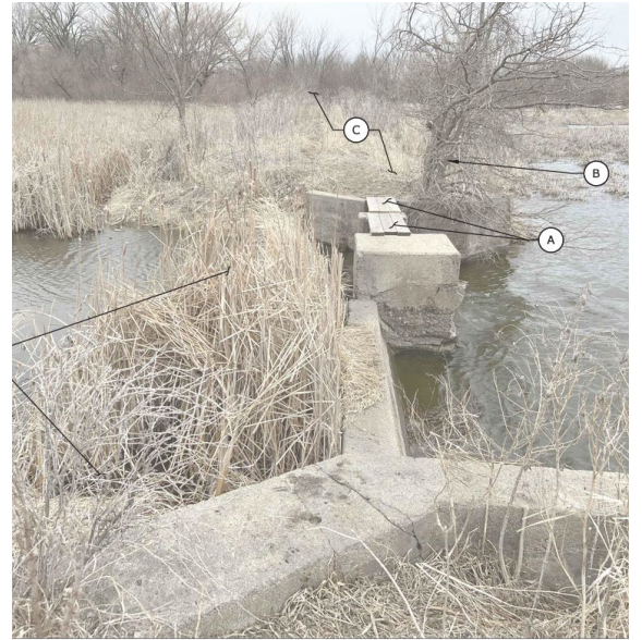
LOOKING NORTH AT EXISTING UPPER STRUCTURE
